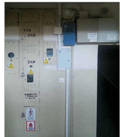
Fig. 5. Photo of completed works - staircase
