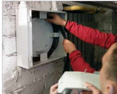
Fig. 2. Works on the arrangement of external cables in MICRO POINT (basement)
